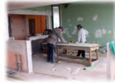
Construction of ICU
