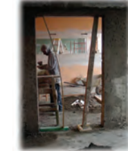
ICU in progress
